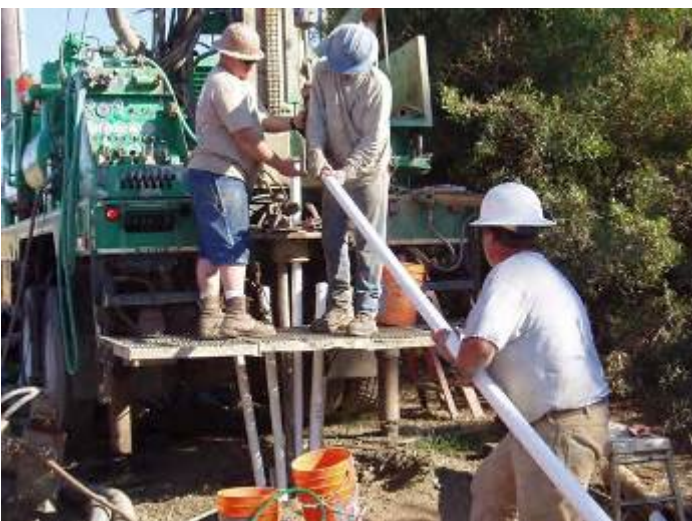
Figure 3C. Installation of 2-inch PVC pipe, which will allow access to specific depths to measure water levels and sample water quality. Note 3 other piezometers are installed already.
