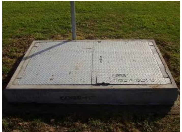
Figure 3E. Typical final installation of 3-by-5-foot, traffic-rated vault. USGS and well ID are welded on top of vault.
