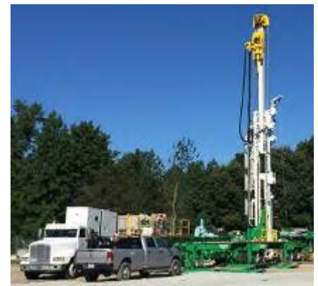
Figure 2. New USGS drill rig will be used to construct the monitoring-well site.
