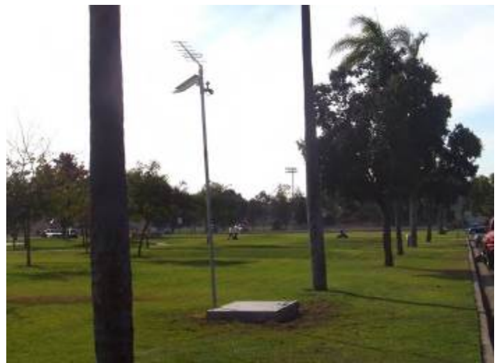
Figure 3F. Final installation of vault, solar panel, and satellite antenna at El Toyon Park, National City, CA.
