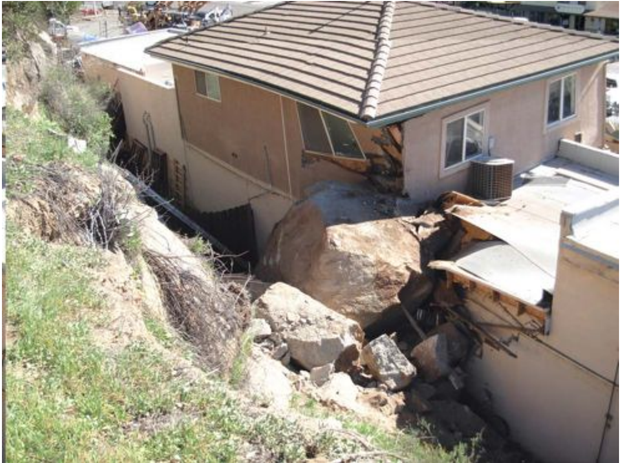
Rock slope failure, Alpine, CA. Cut slopes in granitic rock have an undeserved reputation for being stable.
