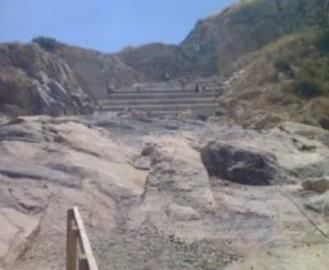
Left: dam and exposed foundation of east end of proposed buttress. SDAG membership for scale. Right: Foundation of proposed west end of buttress, with "stairway" of roller compacted concrete over fractured granitic bedrock. Fractures were pressure-grouted, and weathered rock was blasted away for optimum building conditions.
