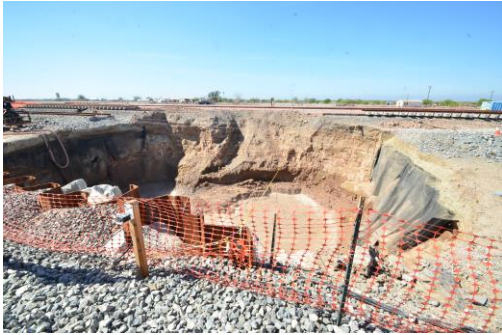
Sinkhole next to Union Pacific railway.
