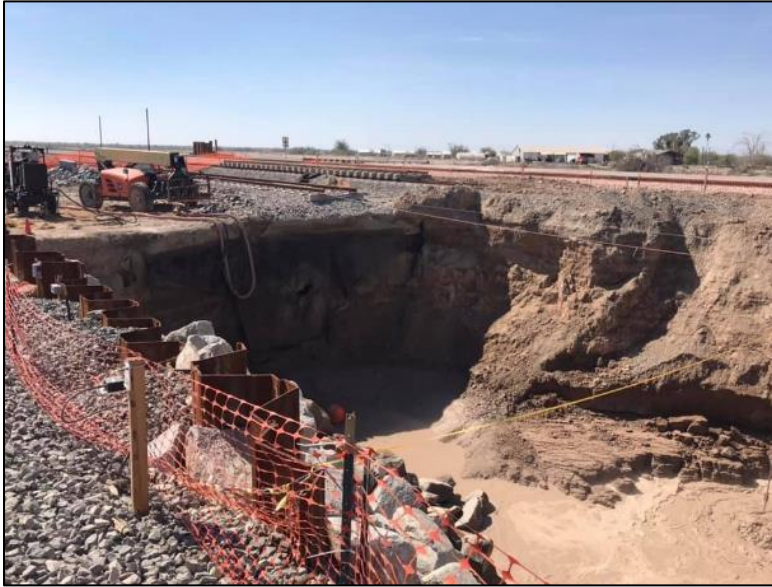
PHOTO 1: Sinkhole next to Union Pacific railway.
